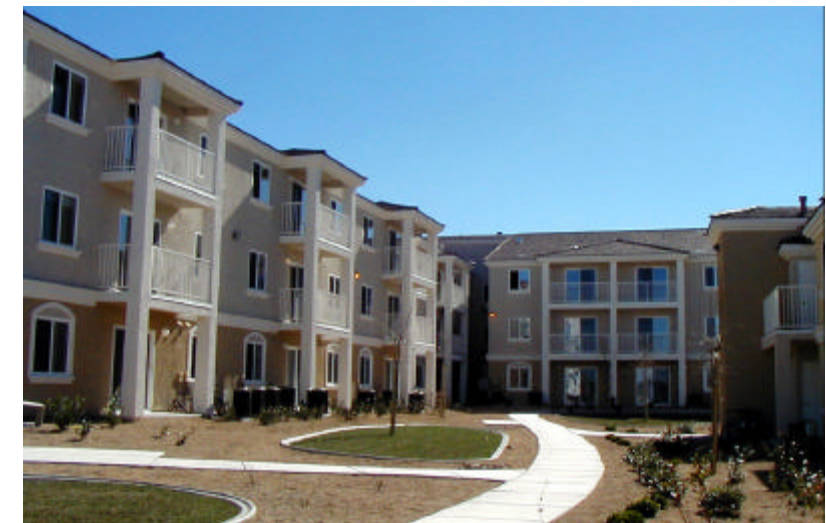
St. Rose Seniors Apartments, dba Vintage at Seven Hills consists of one–two– and three-story buildings of wood frame construction and stucco exteriors and tile roofs.
