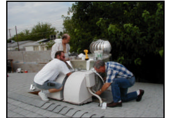
Workers install heating/air conditioning units and insulation as part of the Weatherization Program.
