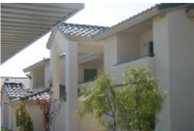
Lindell Harbor Apartments held its grand opening this summer, a NHD tax credit project that provides 19 units of affordable rental housing for seniors.
