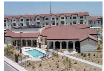
Rear view of Decatur Pines showing desert landscaping
