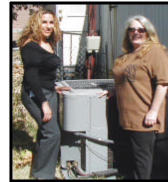
Rita Shaba, of the City of Henderson's Neighborhood Services, inspects new AC unit installed at Debbie Lahn's mobile home. Debbie was homeless before being given the home by the mobile home park management.
