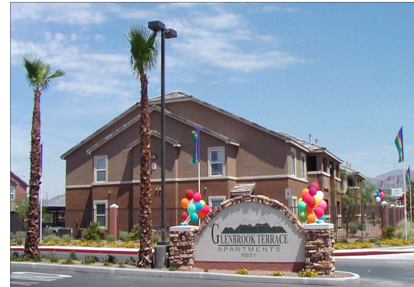
Glenbrook Terrace Apartments
