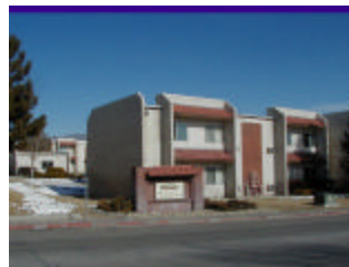
63-unit Horizon Apartments West Wendover, Nevada
