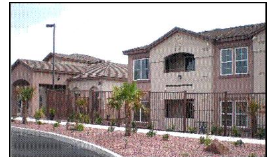
The 238-unit Sonoma Palms Apartments, in northwest Las Vegas, exemplifies the high-quality of energy assurances, passing all the tests and measures verified by an analysis of the building plans pre-construction and verified by inspection and testing post construction using energy efficiency sampling protocol.
