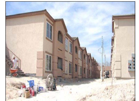
Future 238-unit Sonoma Palms Apartments, located in northwest Las Vegas
